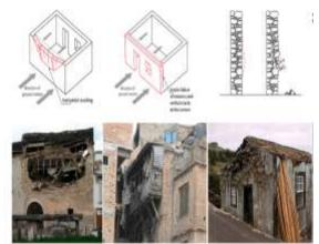
Various types of failure in masonrypier:-(a)sliding shear (b)rocking (c)diagonal shear cracking
